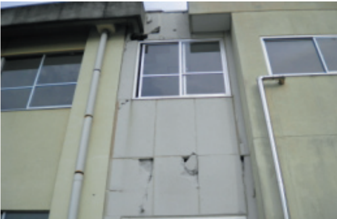
Cracked wall 3/11
