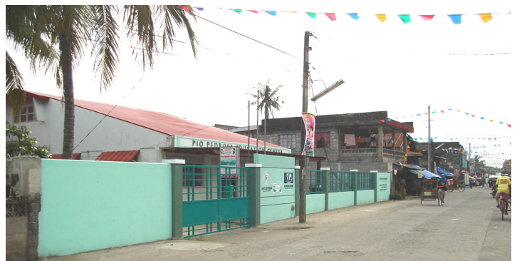
Shown here is the full length of the completed front CHB fence along F. Montejo St. taken from the south end of the fence.
